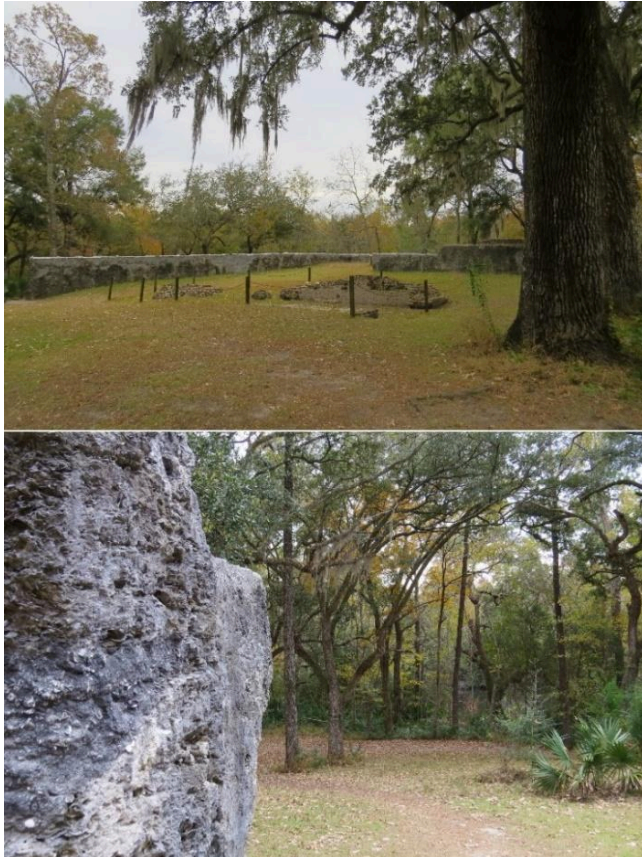
Figure 5. Remains of Fort Dorchester. (Top) View within the tabby walls of the fort with brick remains of the powder magazine in the middle. (Bottom) Closeup of the tabby wall with Ashley River just beyond the clearing. Tabby was made from a mixture of lime, sand, and oyster shells. (C. Leon Harris)
